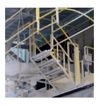
**LISTENOW** supplies **LIS-klap** safety folding steps with 3, 4, and 5 steps to give operators easy access to vehicles, such as tankers, silo trucks and tank wagons.
